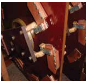
TLH-21 Moveable Contacts in Bridging Positions
