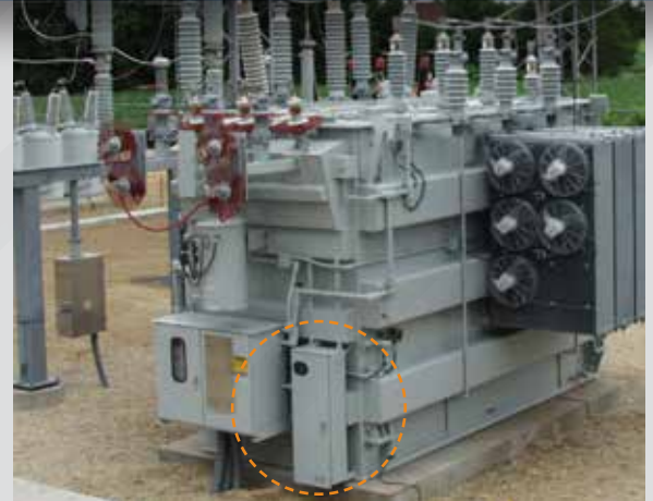
Supply and tank pressure gauges on the Inert Air System are easily viewed through a large viewing port on the cabinet door.
