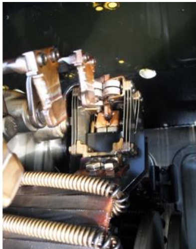
Film on Selector Switch Contacts
